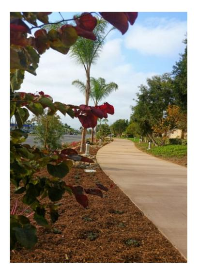
The improvements to the trail, which spans the west side of Harbor Boulevard between Fair Drive and Merrimac Way, consisted of the removal of the old asphalt trail and concrete sidewalk, and construction of a 12-foot wide, colored concrete multipurpose trail.
