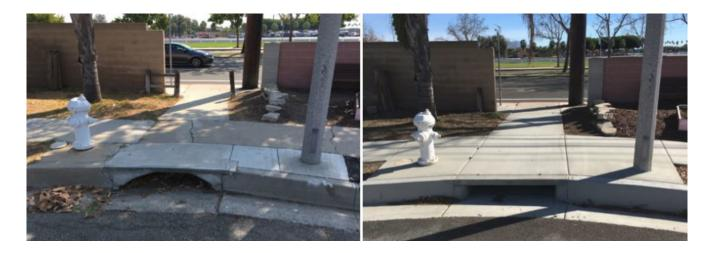
Public Services also recently completed the reconstruction of the parkway drain at Wellesley Lane near Fairview Road (see before and after photos). The project entailed demolition of the deteriorated parkway culvert and reconstruction of a parkway drain to meet the city's standards. In addition to improving drainage conditions in the cul-de-sac, the project also included minor improvements to deteriorated sidewalk to eliminate displacements.
