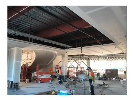
The installation of insulation and drywall is almost complete and ceiling systems are currently being constructed. Windows and storefronts are being installed, the elevator shaft is in place, and exterior scaffolding is erected for surface treatments.
